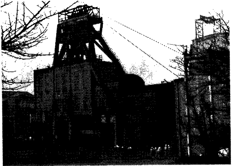
Harworth No.1 pit-head
