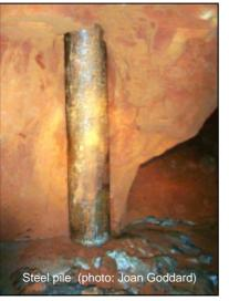
Some of us (not me!) climbed part way up another shaft which had two horizontal brickarched, flagstone-paved passages leading off it. Modern features we saw were massive concrete foundation pillars and steel piles to support buildings above the mines.
