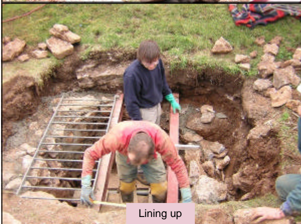
Lowering the RSJs into position
