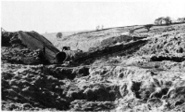
PLATE VIII. Installation of flood channel, Mendruch. Photo: R. Agard
