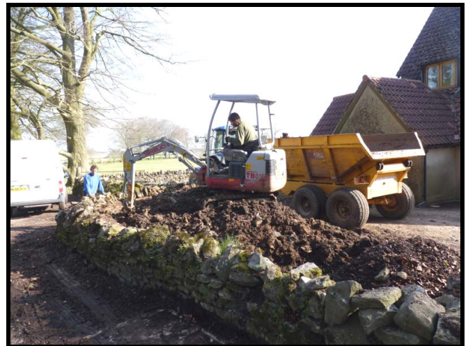
Biff and Buddy working on the car park. Photo: Mark Ward
