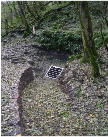
Photo 5. Drystone wall, dam and new gate/grill at Longwood Valley Sink, 30 th Oct 2013 [Photo: Joan Goddard]
