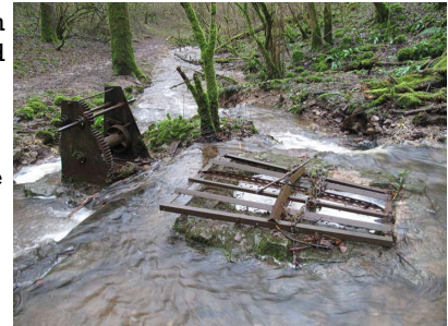
Photo 1. Before work started. Water overflowing Longwood Valley Sink and continuing down the valley [Photo: Alison Moody]
