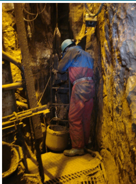
Dave Turner working on the 166ft platform winching up spoil from below
