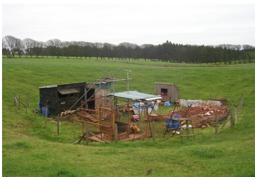
Photo 10. Home Close Hole dig site with Engine House to left of picture [Photo: J.Goddard, Dec 2013]
