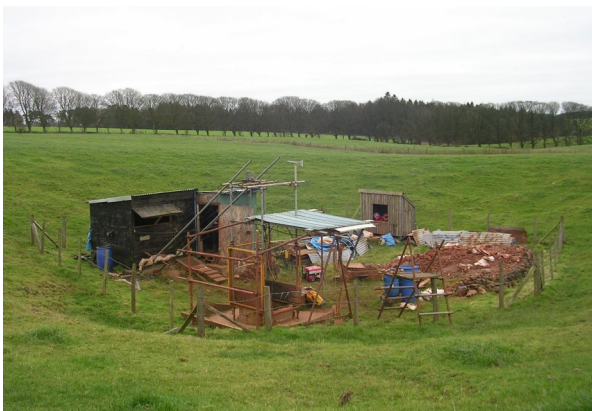
Home Close Hole dig site with Engine House to left of picture [Photo: J.Goddard. Dec 2013]
