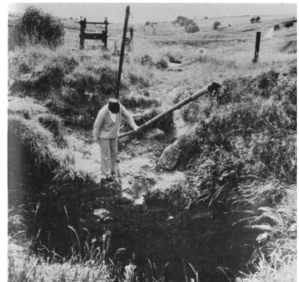
Photo 3. The swinging jib at Blackmoor (Stainsby's) Shaft. Note old winch in the background, pre April 1972 [from 'Britain's Old Metal Mines' by R.H.Bird]
