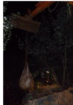
Lifting with the digger by Estelle Sandford
