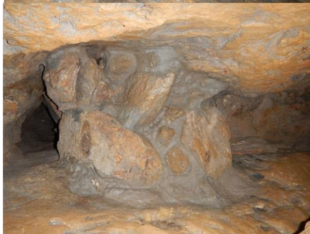
Right Bottom: The same boulders, post stabilization.
