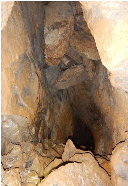
Left: Looking along passage with the boulders that had been held up by a now disintegrated Stemple.
